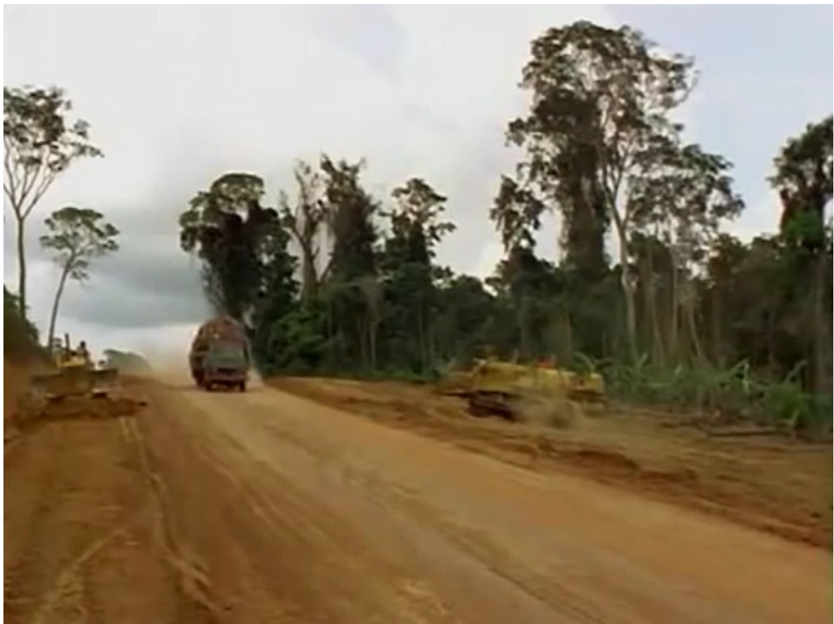
Figure 3. The Caravana and the Caterpillar bulldozers.
