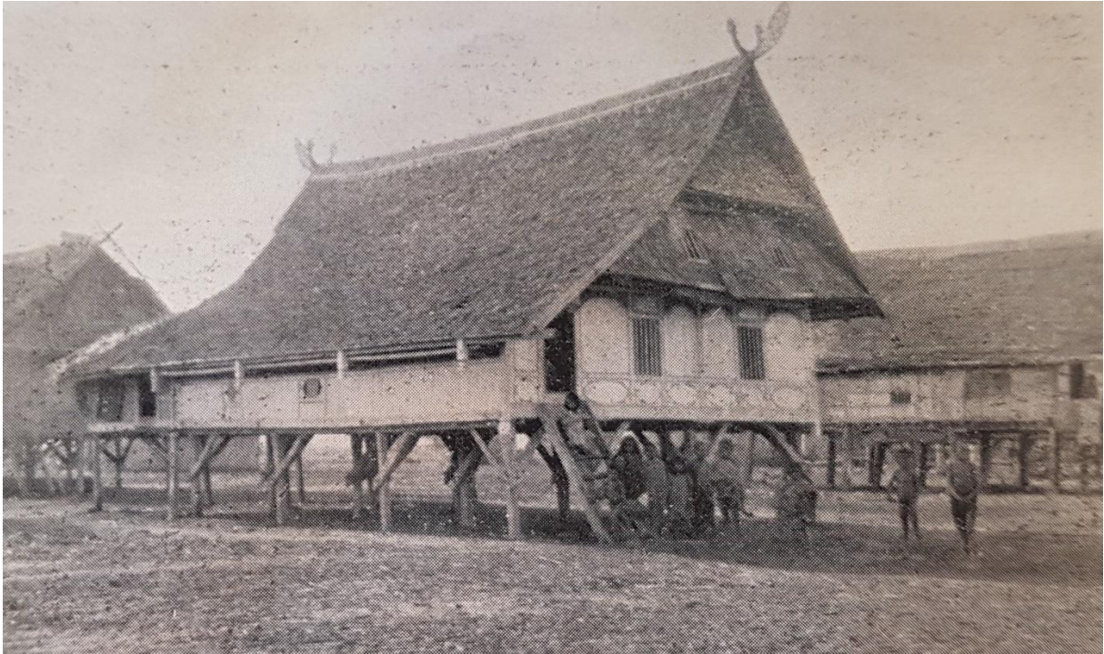
Image 8 House in the department of Goa, Zuid-Celebes. The houses were built on poles, and consisted of bamboo, palm-leaves and other wood. 270
