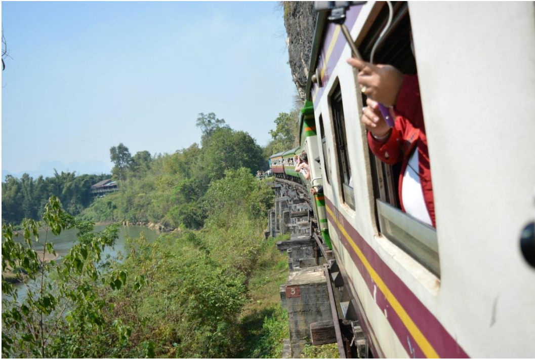
Figure 42. The train crosses the wooden Tham Kra Sae Bridge
