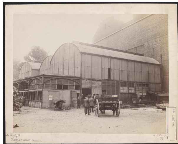
Figure 4: The Brompton Boilers (collections.vam.ac.uk)
