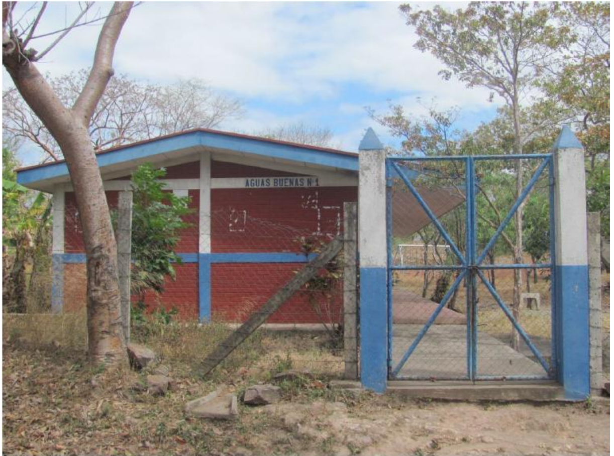
Figure 15 Primary school in the community of Aguas Buenas 1. Photograph taken by Eva van Dosselaar, January 2016.
