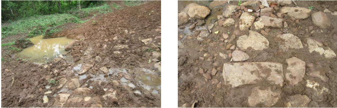
Figure 28 and 29 The use of uncarved monoliths to harden muddy passageways is illustrated in these photographs. Photographs by Anne Vera Veen, June 2016.
