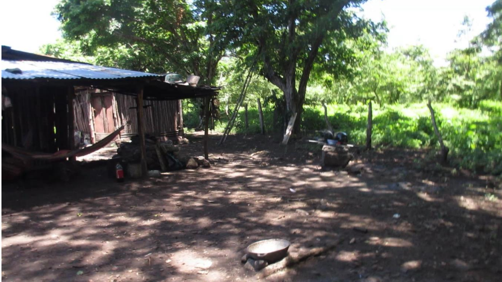
Figure 13 Small residence in Santa Rita. This house is constructed directly on the stamped earth. The walls consist of wooden posts. For the roof, metal corrugated sheets are used. Photograph by Anne Vera Veen, June 2016.
