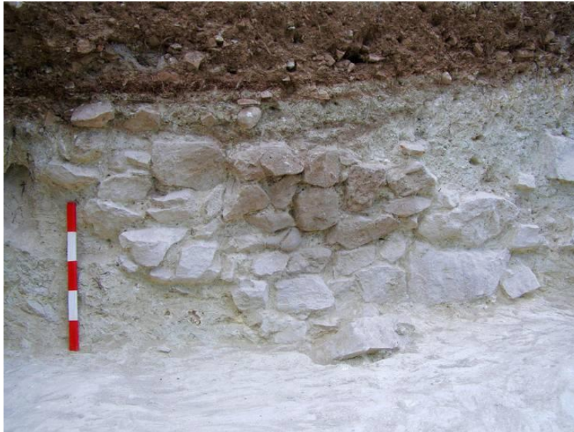
Figure 16: Area TT, Wall 4, view from the west; the darker stain on its face indicates the position of the pit represented by SU3-4 (photo: author)
