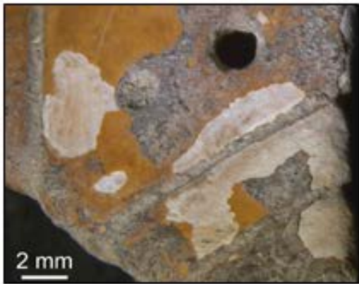
a. Erosion of upper layer of shell and dirt attached to the surface (VA14019)
