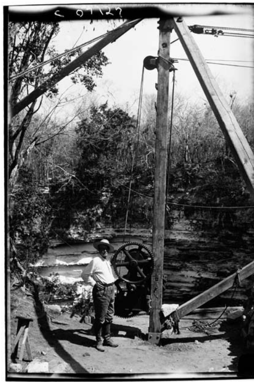
Figure 8. Thompson standing next to his device to haul in the buckets from the dredge (from the online collection at www.peabody.harvard.edu ).
