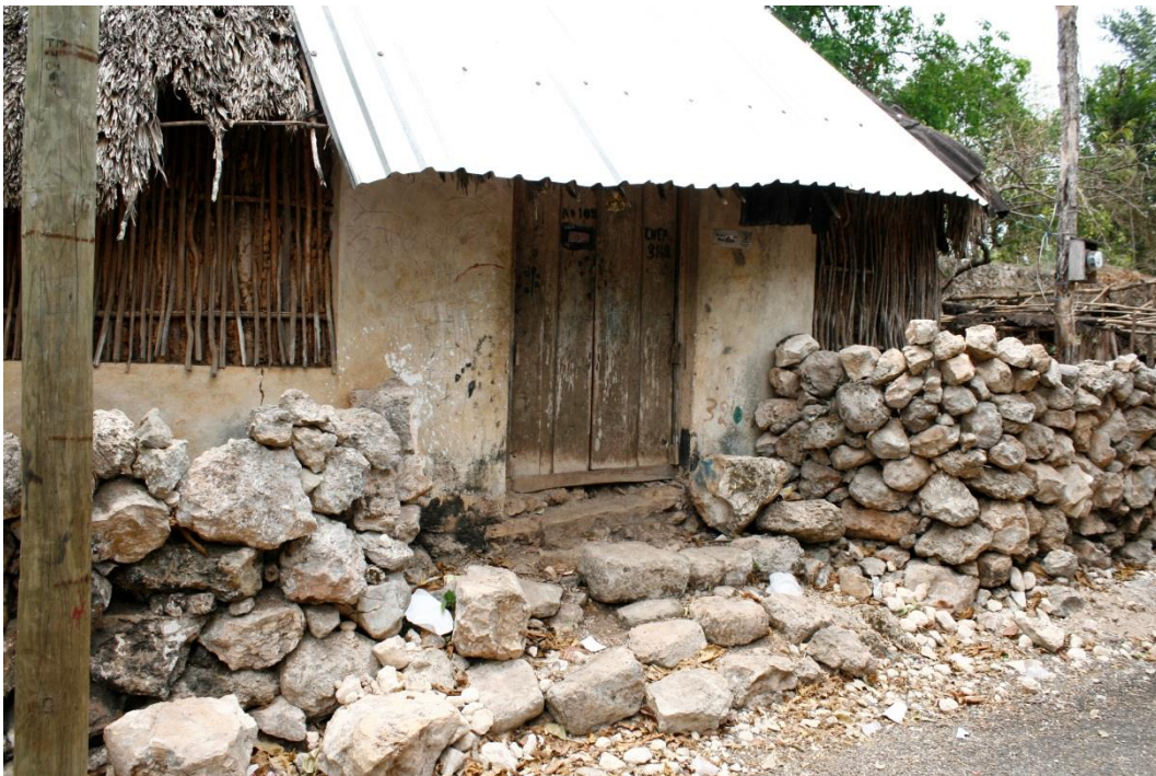
Figure 16. An interesting mix of building traditions: a base of concrete, the traditional Maya wooden and clay walls, thatched roof partly covered with corrugated iron
