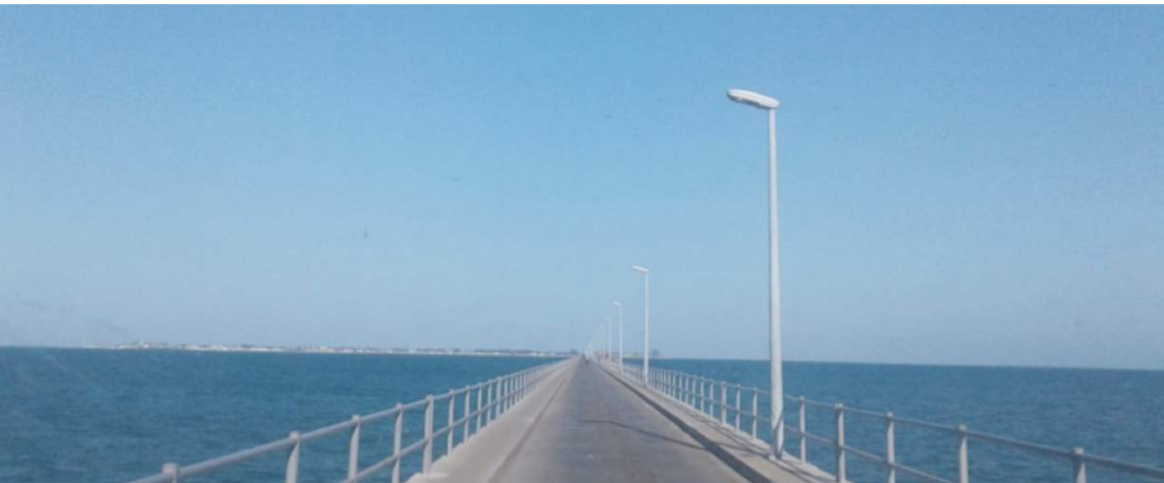
Bridge from mainland Namputa to the Island of Mozambique. Photo Miriam Ocadiz Arriaga
