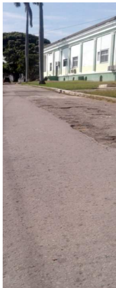
View of the Hospital Salvador Allende in Havana at midday.
