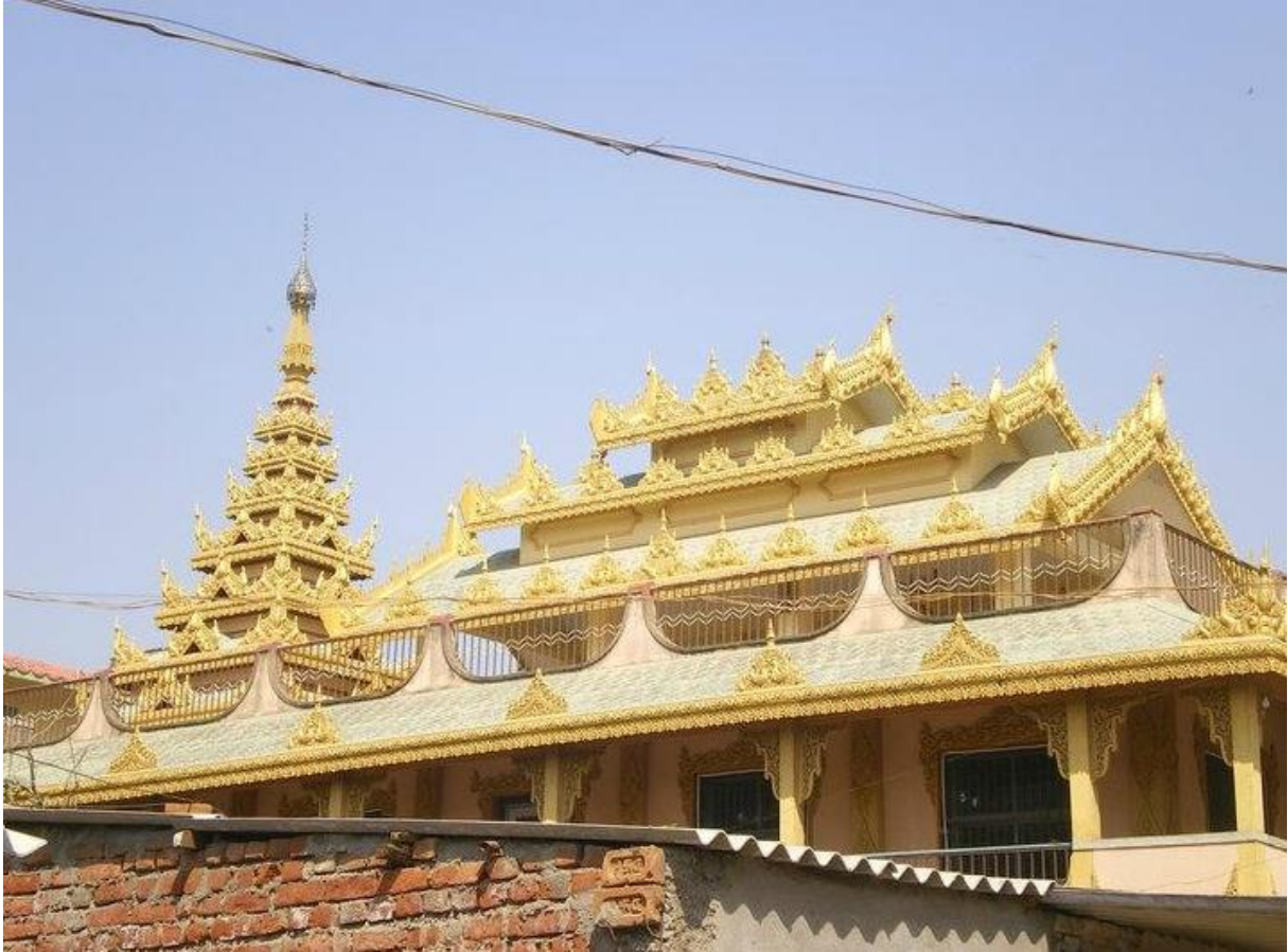
Figure 6. The roof of the Burmese Temple.
