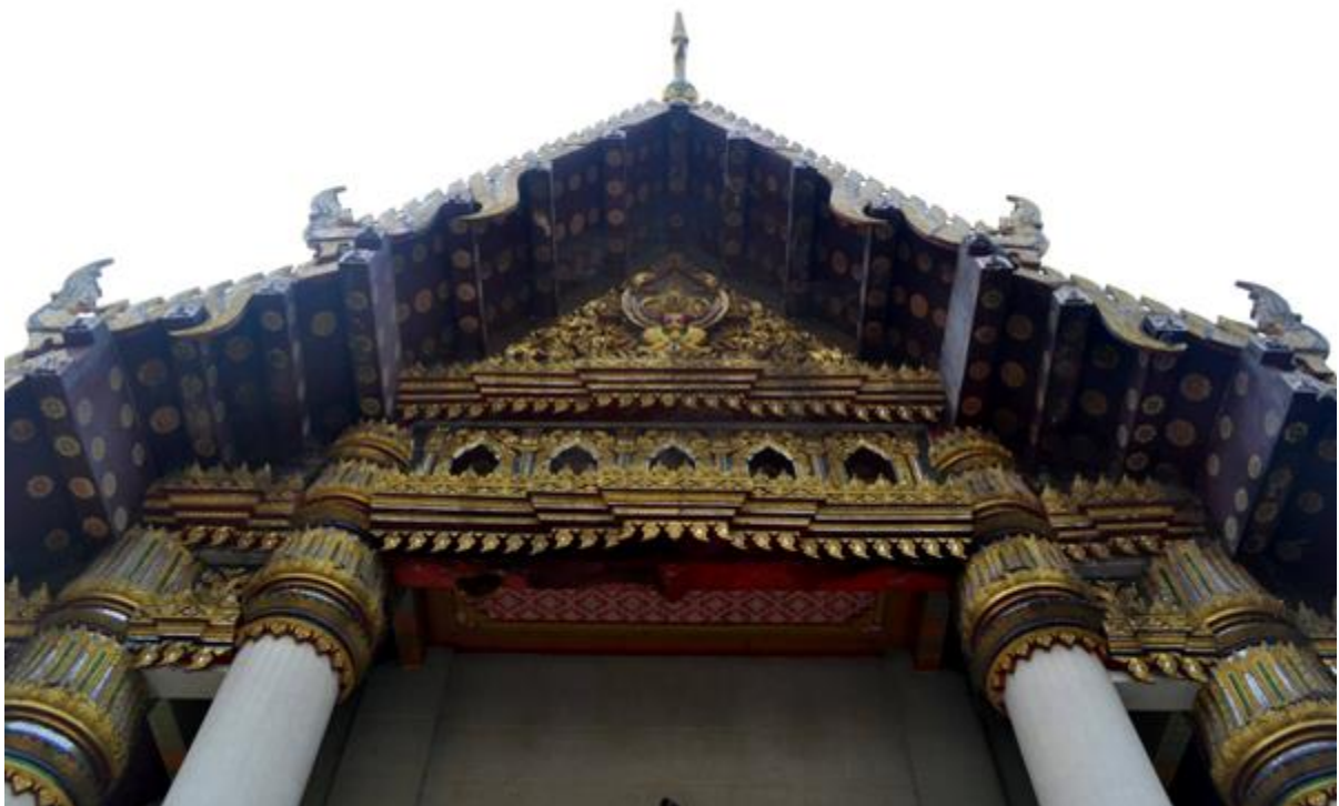
Figure 34. The rooftop of the Thai Temple with a seal underneath the top.
