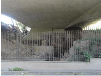
Figure 10: Fly-over bridge with fenced-off ruins (own photo)
