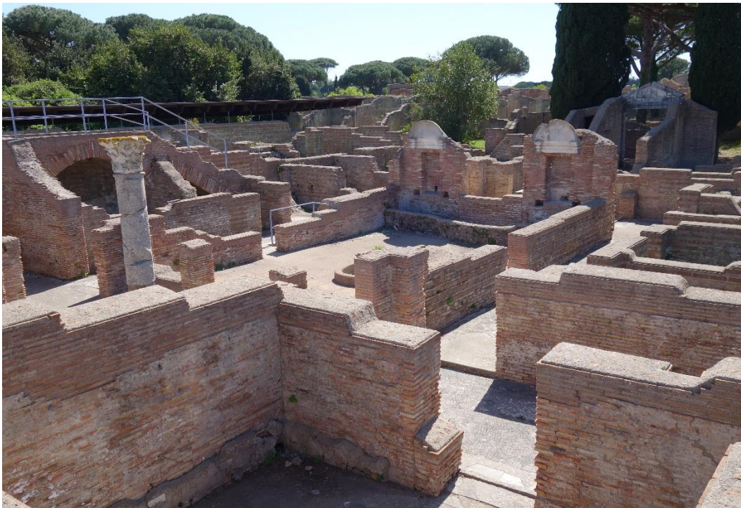
Appendix H6: Overview the back half of building V ii 4-5 (by author).
