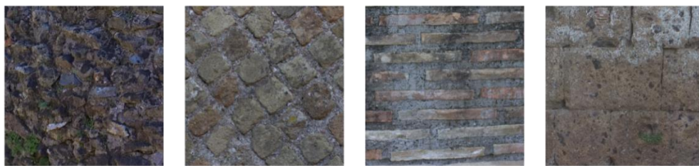
Figure 19: Illustrative examples of the different construction techniques based on examples from Ostia Antica. From left to right: opus caementicium, opus reticulatum, opus vittatum and opus quadratum (Brunke 2017).
