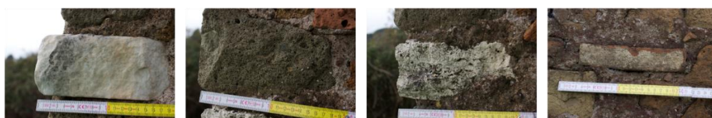
Figure 30: Overview of new materials in the tambour. From left to right: marble, peperino, travertine and bricks. Plates 4 and 5 provide information about the distribution (Brunke 2017).
