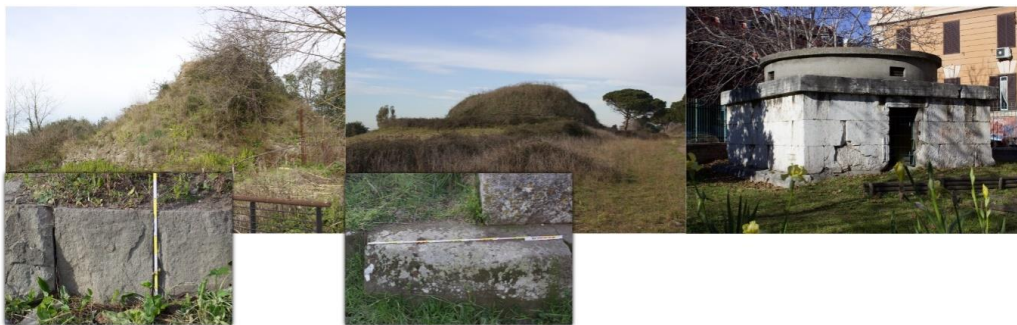
Figure 27: Similar tumuli with partly intact casing of opus quadratum along the Via Appia (left and central) and in Rome (right). The casing is of peperino and travertine and the individual blocks are about 50-60 cm high (Brunke 2017).
