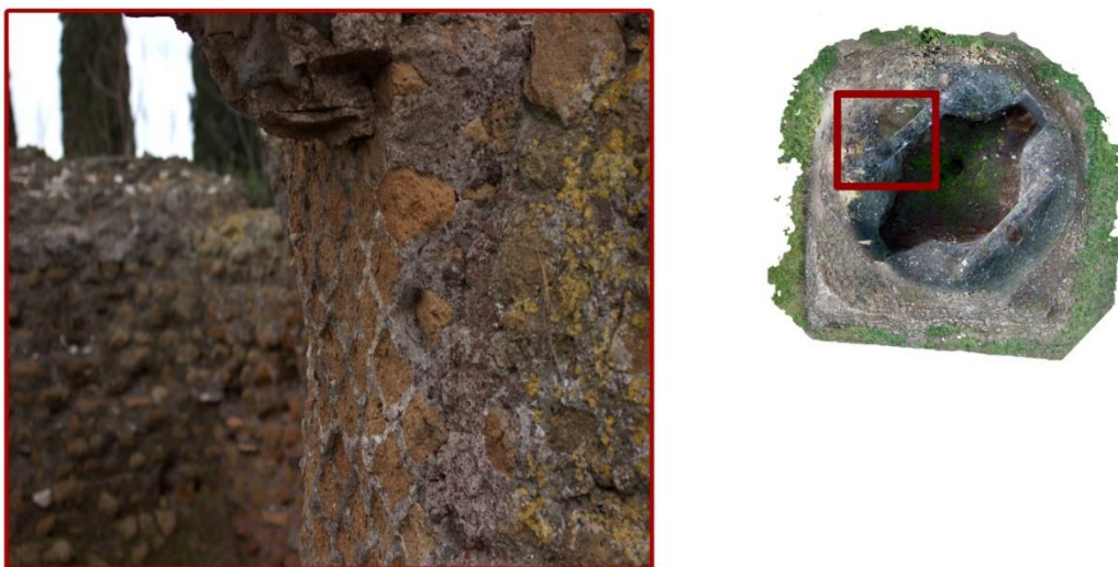
Figure 34: Part of the opus reticulatum on the inside of the monument (Brunke 2017).
