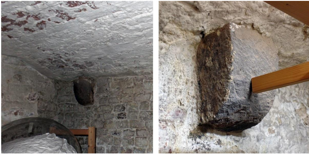
Figure 2.4 Photo of remaining corbels in cellar D8a (Brink 48) just below the current vaulting (source: photographed by author).
