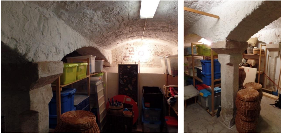
Figure 7.8 Example of a cellar of the Deventer type (under Brink 48), including columns of Bentheimer sandstone (source: photographed by author).
