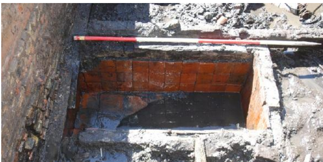
Fig. 6.1: Example of an early cistern at Rozenstraat 72 , with glazed tiles on the walls and floor (Gawronski and Veerkamp 2011, 53).
