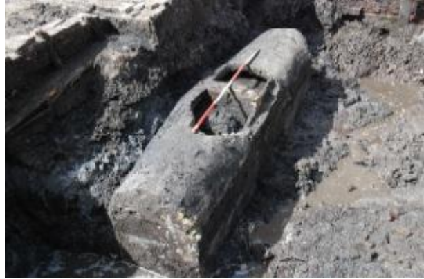
Fig. 4.3: Cistern at Elandstraat 103-105, equipped with two shafts in the centre (Gawronski et al. 2010, 23).
