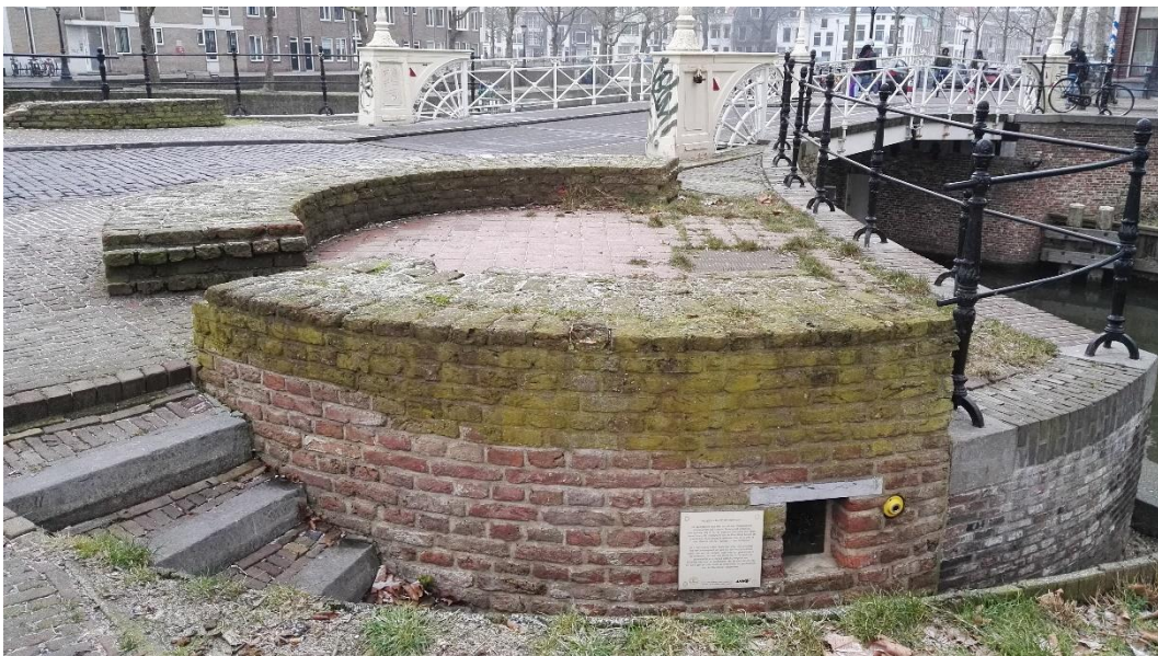
Figure 41, the reconstructed front towers of the Weerdpoort with an added window to look inside.
