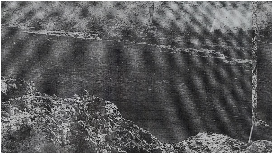
Figure 13, the brick retaining wall standing over 2 metres high at the excavation on the Nieuwe Kade, after De Groot 1989, 132.
