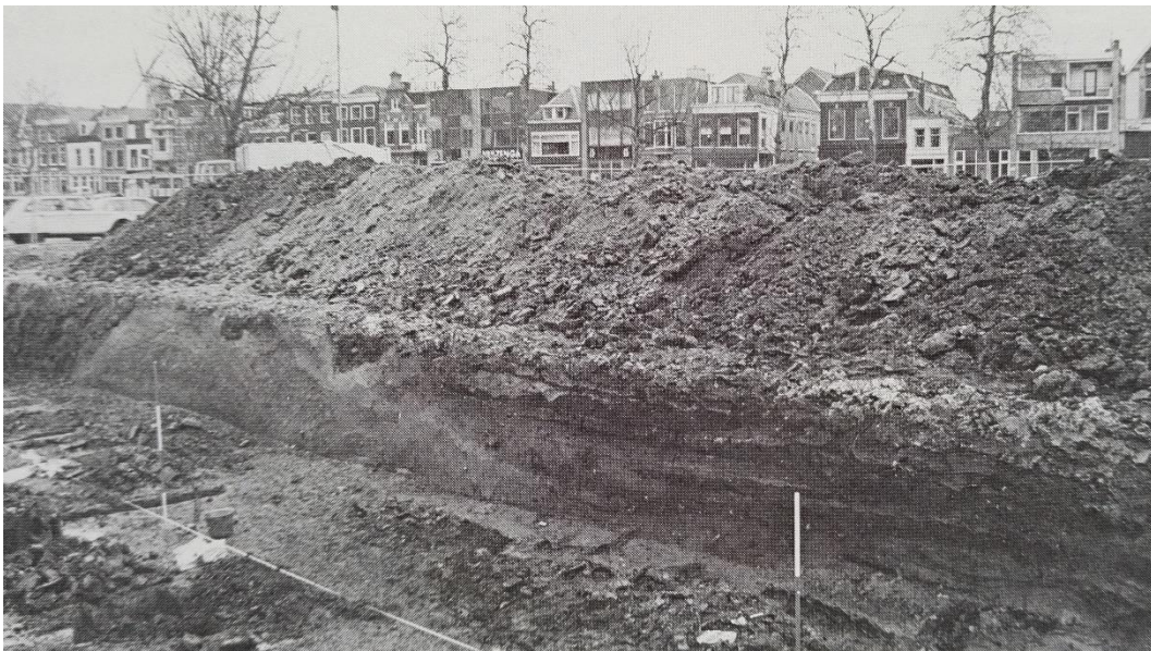
Figure 15, profile in which the earthen wall at the Jan Meijenstraat can be seen (left). After De Groot 1981, 49.
