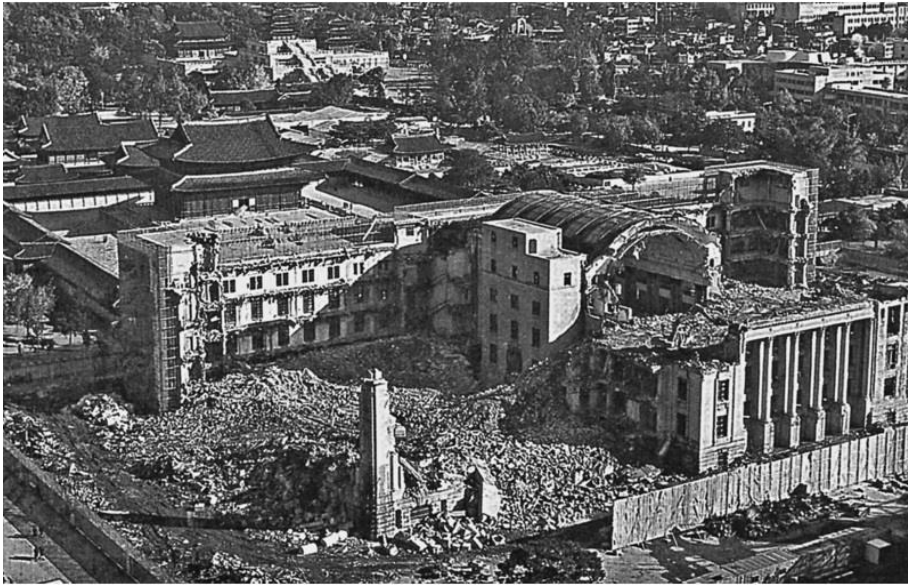
Figure 6. Demolishing the Government-General building, 1995
