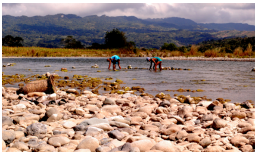
Figure 11 – Fishermen building a dam Photo by K. van Lieshout (2013)
