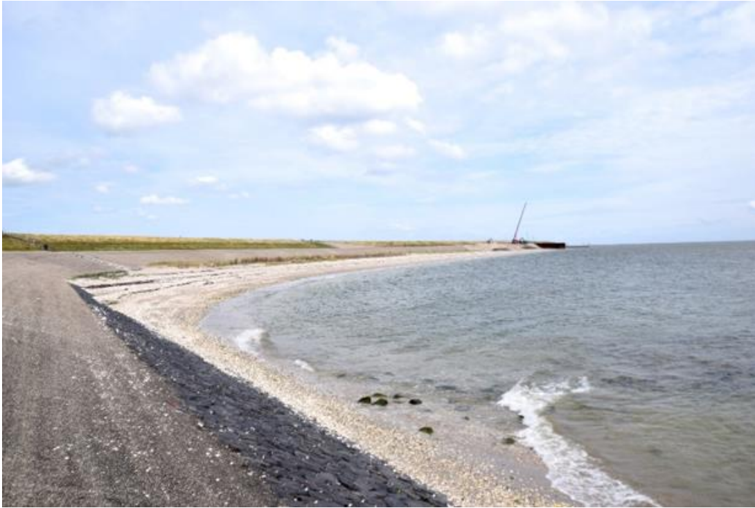
Picture 16: Ceres Beach as seen from its most northern point, the dyke construction works are visible in the background.
