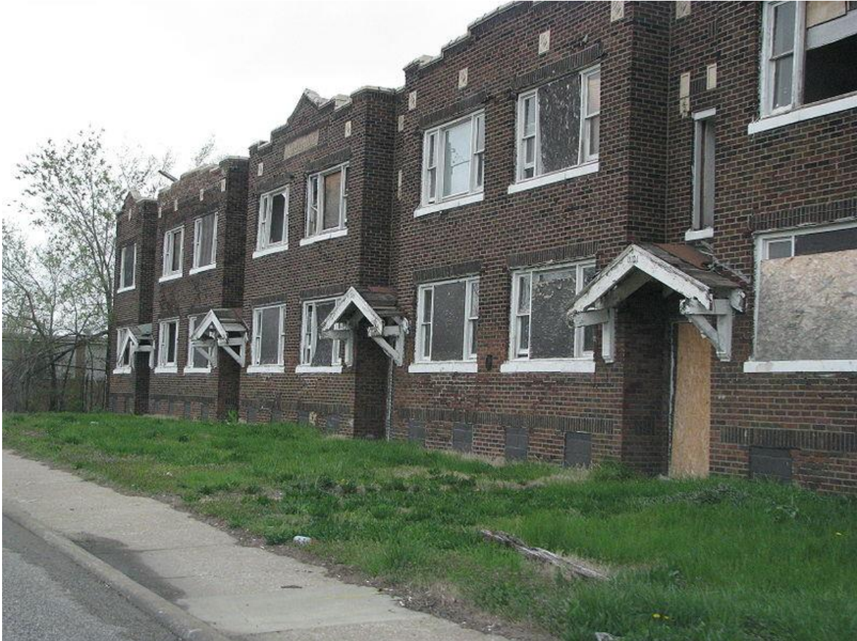
Fig. 3: 2008 photograph of abandoned apartments in East St. Louis. 141
