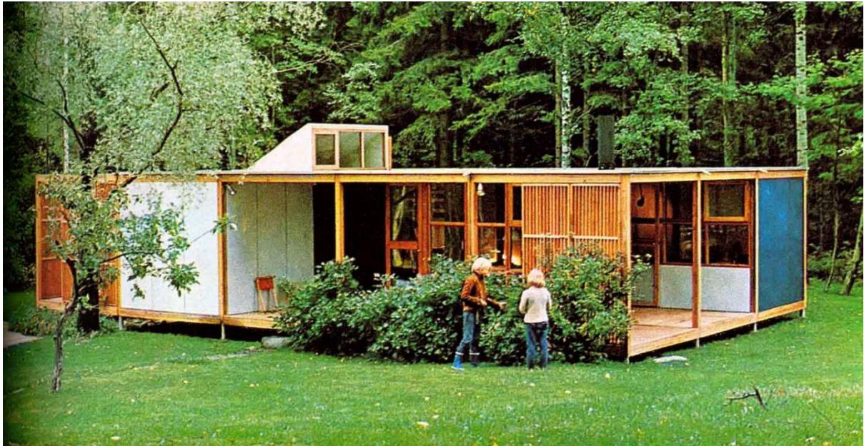
Fig. 91 – Juhani Pallasmaa and Kristian Gullichsen, The Moduli 255 Summer House System, 1968-72. Retrieved from https://proyectos4etsa.wordpress.com/2011/11/07/sistema-moduli-kristian-gullichsen-y-juhani-pallasmaa-finlandia-1968/ on 15 May 2016.
