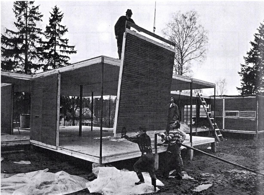
Fig. 22 – Raimo Kallio-Mannila and Teuvo Koivu, The construction of the Domino System , 1964, place unknown. Source: The exhibition catalogue 'Exhibition of Finnish Architecture', The Hague April 28 – May 19, 1975, Netherlands Congress Centre, Turin 1973-74.
