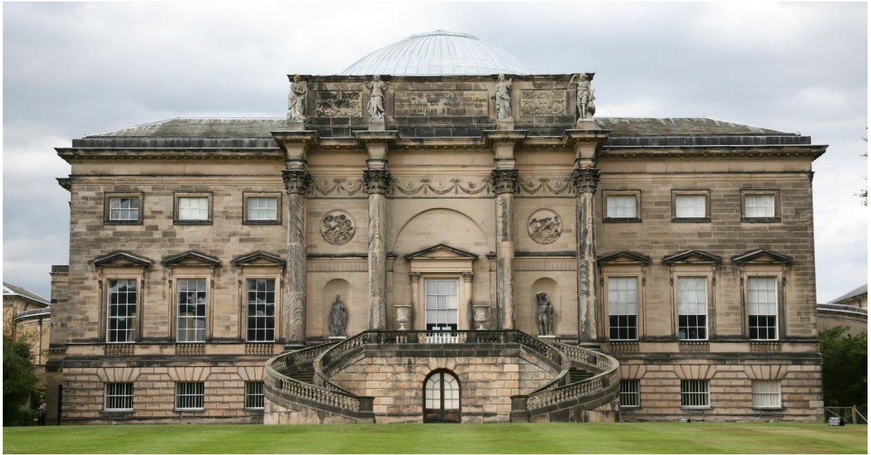
Fig. 21: James Stuart/Matthew Brettingham the Elder/James Paine/Robert Adam, South façade of the main building of Kedleston Hall, 1759
