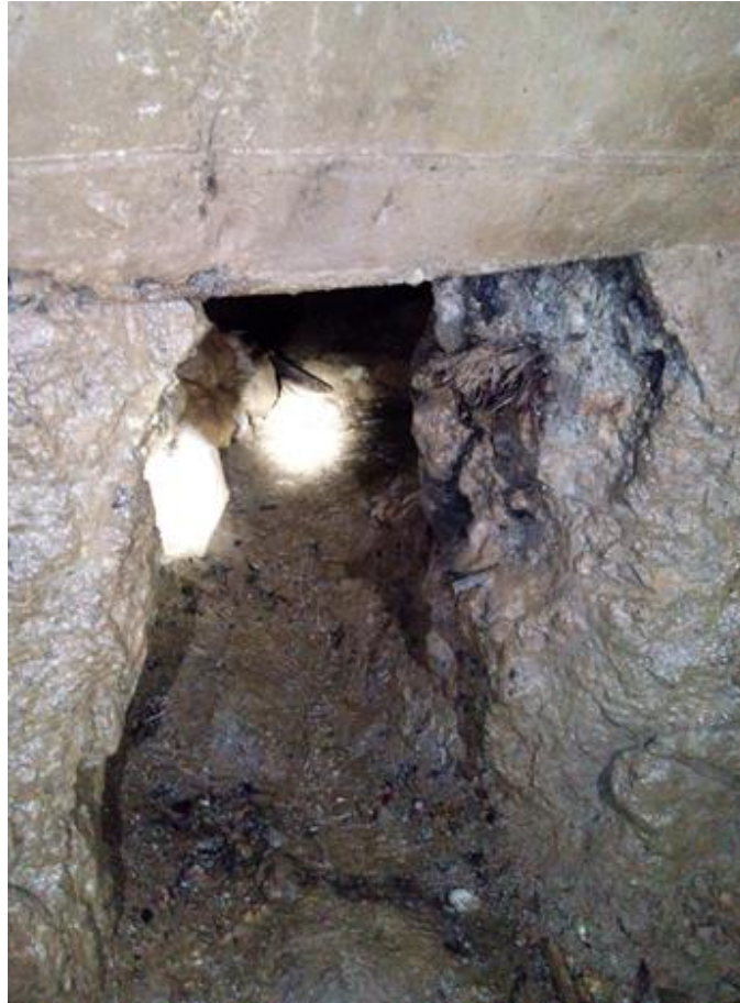
One of the many other tiny holes along the main tunnel that serves as entrance to a work area
