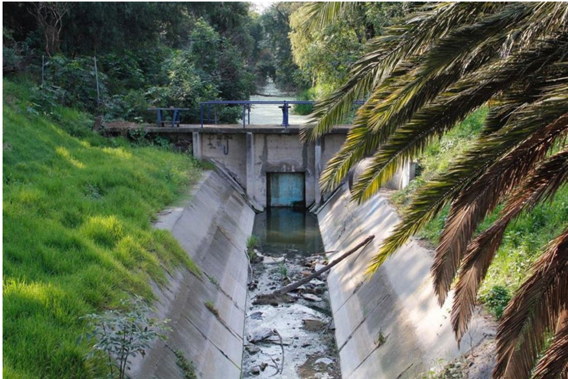
Fig. 8. Contemporary view of Canal Nacional, Mexico City.
