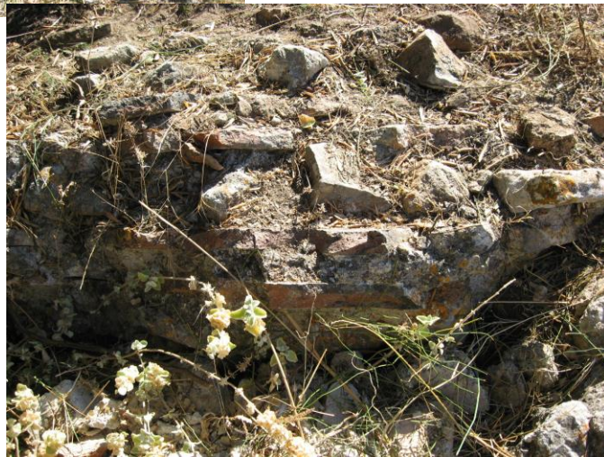
Figure 3.10 (right): Close-up of feature E, the large bricks are clearly visible, as well as the caementa . (Photo: Yannick Boswinkel 2011)
