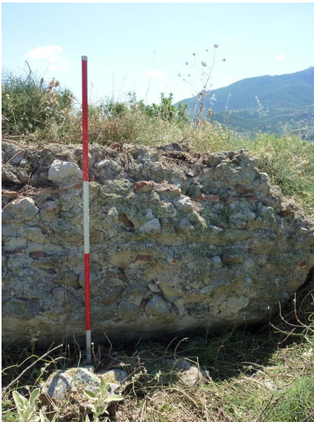
Figure 3.4: Feature B. Note the curve inward at the bottom, which is also plastered. (Photo: Hanna Stöger 2011)
