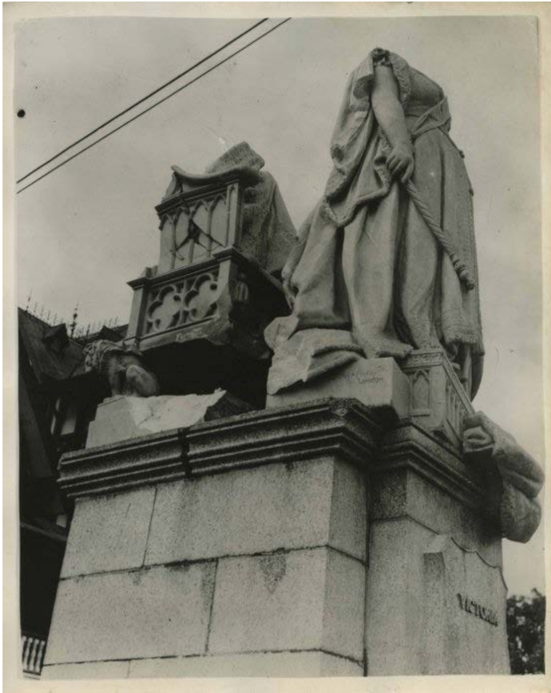
Figure 32 Damage to statue of Queen Victoria due to dynamite explosions 1954.
