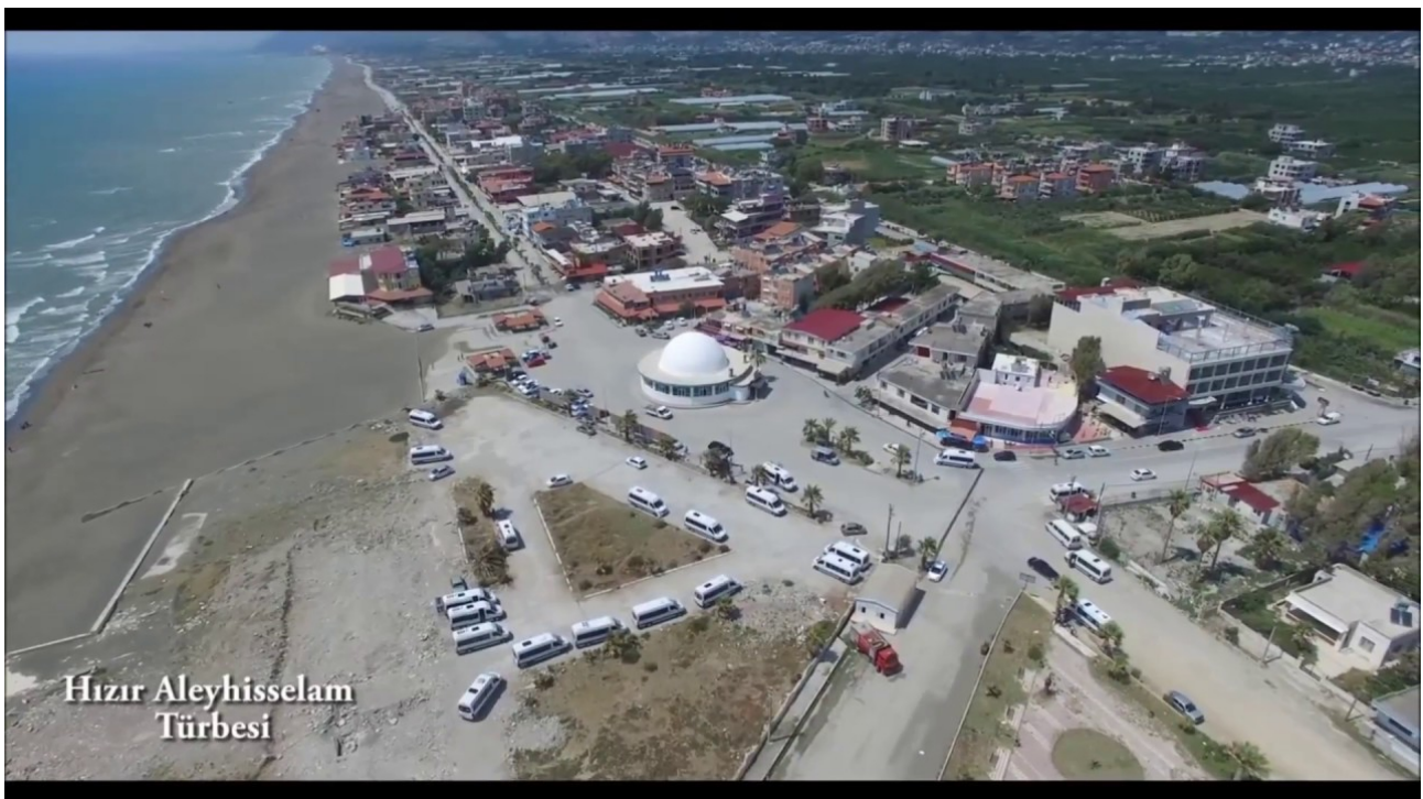
Illustration 13: The Deniz Sitesi and the Hızır site before the broader renovations.
