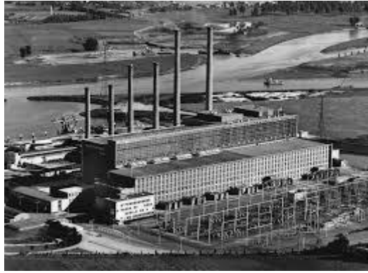
Figure 4.2: Maascentrale Power plant in operation (ca. 1978)
