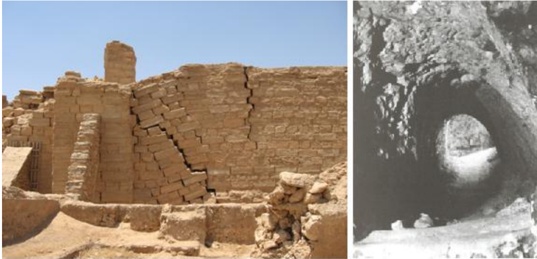
Figure 18: Left: Breach in the city wall at Dura Europos, Syria due to mining activity. Right: A mine-tunnel at Dover Castle in Kent associated to the siege of 1216 (After Wiggins 2003, 16).
