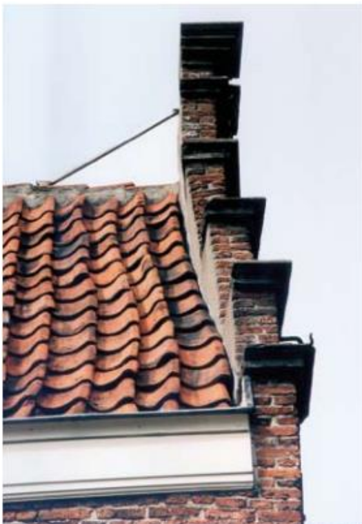
Figure 7: In 1466 a new type of tiles came into use in Holland, the “Zwolse Quakpan”, whose design quickly became known in Dutch as the “ gegolfde holle pan ” which is depicted on the image (Polman and van Rooden 2008, 2).
