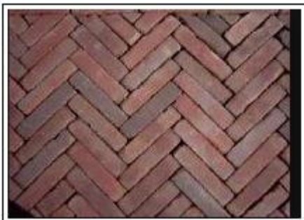
Figure 24: Keperbond, present as a floor in the castle of Huis ter Kleef (After Werkspot 2009).
