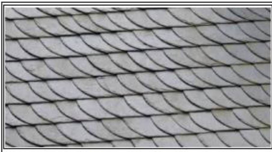
Figure 8: These slate tiles, which are formed into a scale like style (Boeder and Tolboom 2010a, 1).
