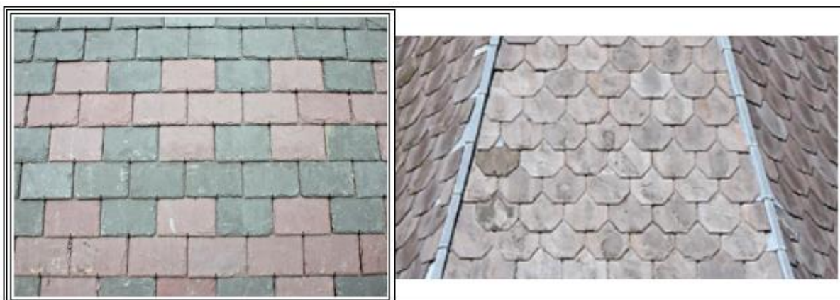
Figure 9: Two different forms of square slate tiles (After Boeder and Tolboom 2010b, 1-3).
