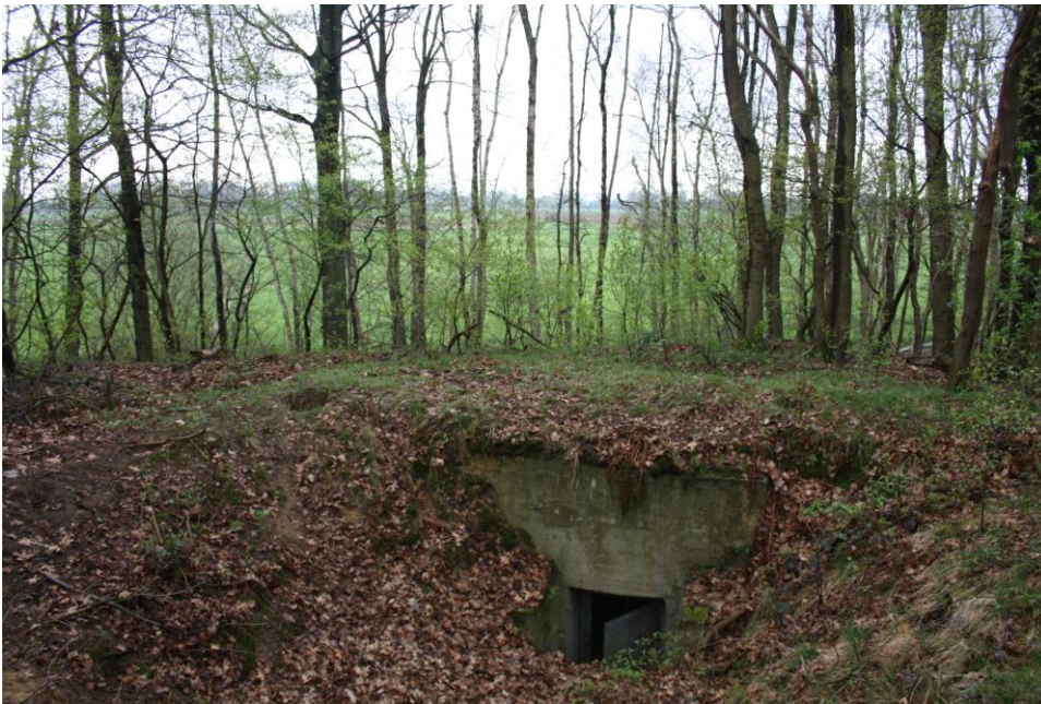
III.1: Betonnen MG bunker.
