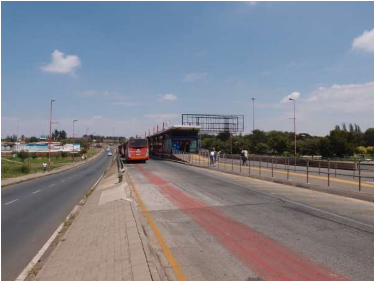
Figure 2: Rea Vaya station Thokoza Park in Soweto 103
