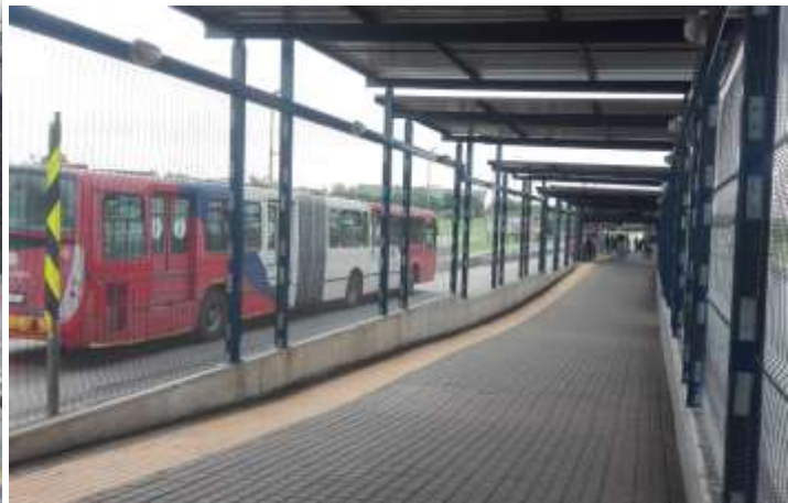
Figure 8: Thokoza Park Station 328
