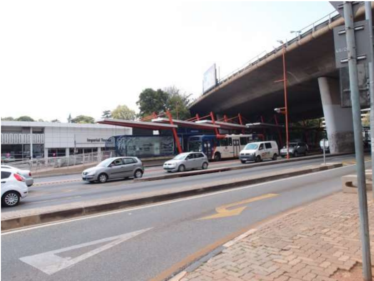
Figure 6: Rea Vaya station Wits Station 246
