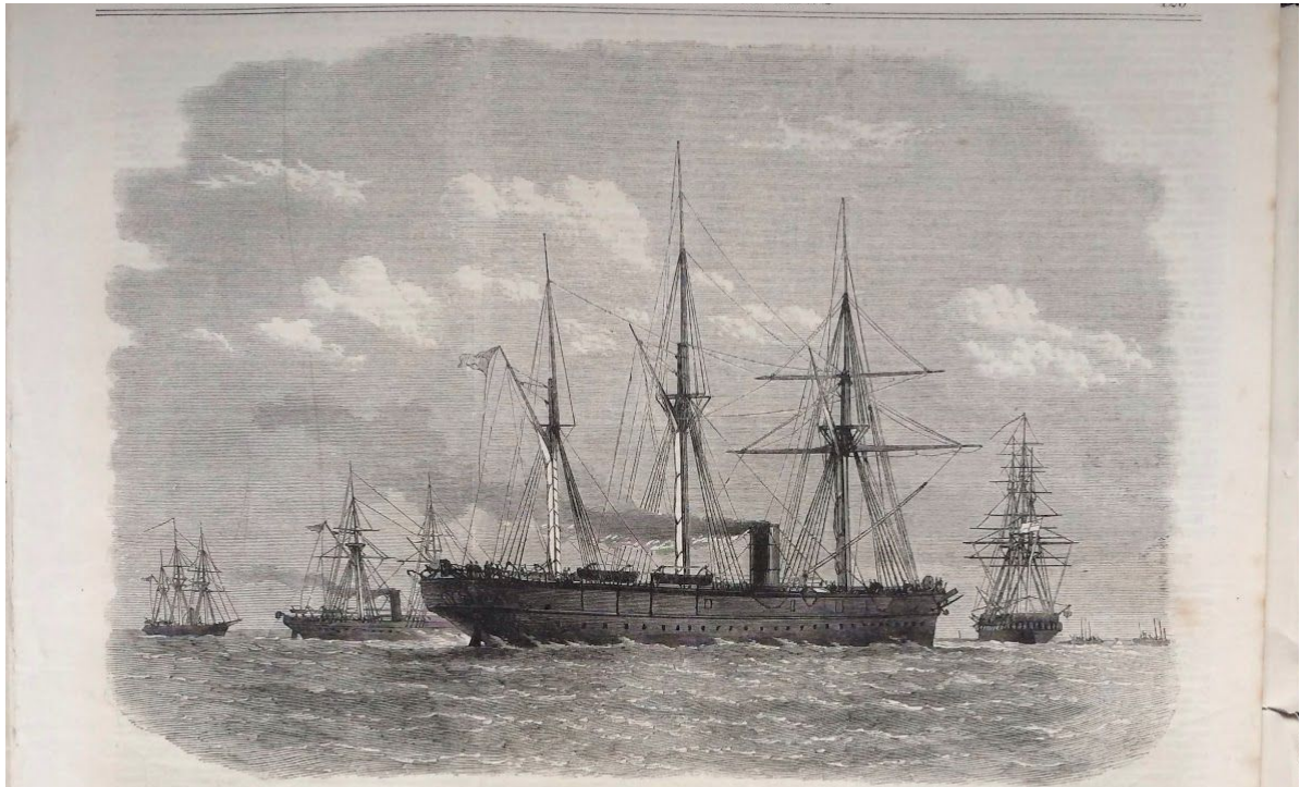
LAYING THE SUBMARINE CABLE BETWEEN MALTA AND ALEXANDRIA.
