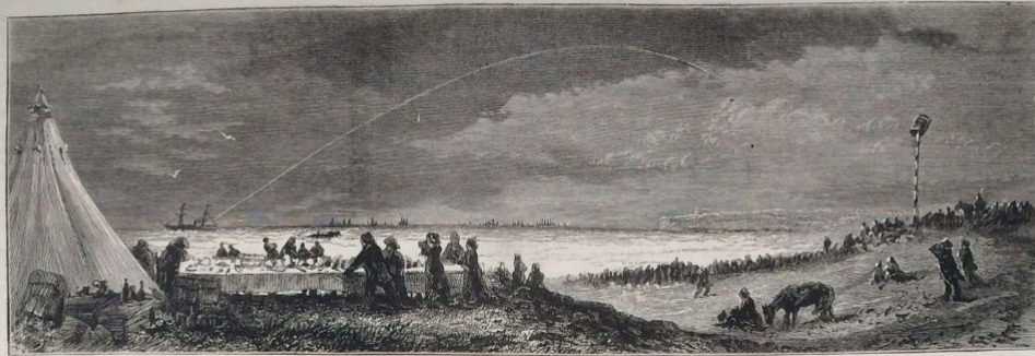
LANDING THE SHORE END OF THE SUBMARINE CABLE NEAR DURBAN, NATAL
