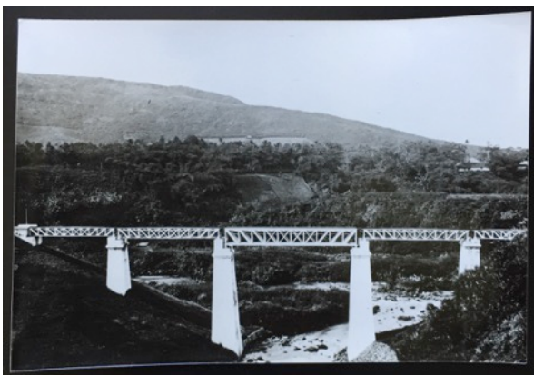
Fig. 48: Recto: Bridge, b&w photograph, paper, 12.9 x 8.8 cm, without further information.
