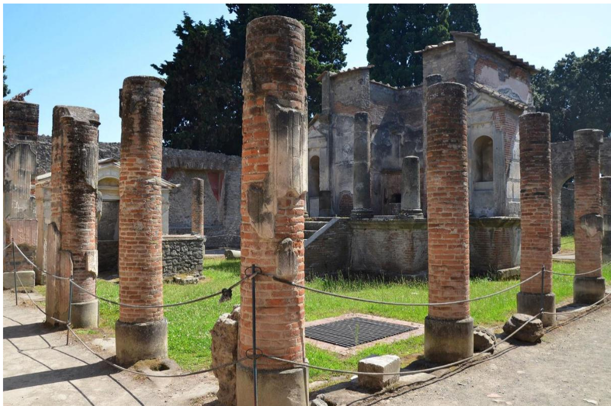
Fig. 3.33: The shrine of the Temple of Isis at Pompeii surrounded by the columns of the portico. It is possible to see the bricks that were employed in the construction of the temple by looking at the columns (www.ancient.eu)
