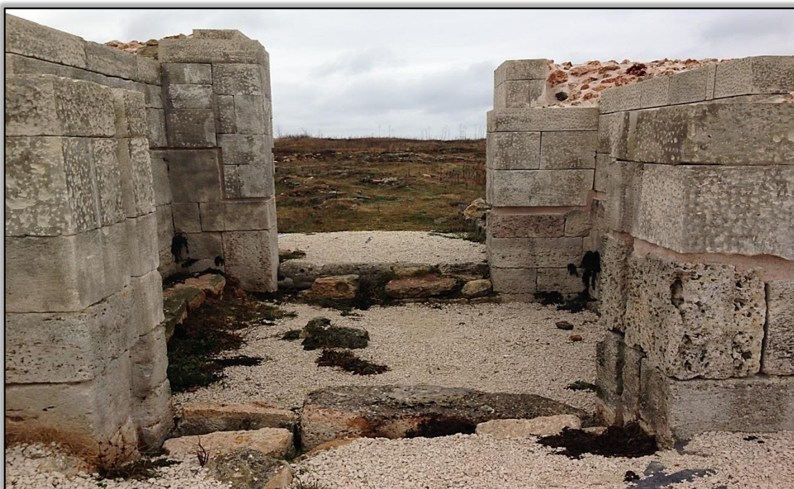
Fig.9. Restoration of the Western tower gate (photo by the author).
