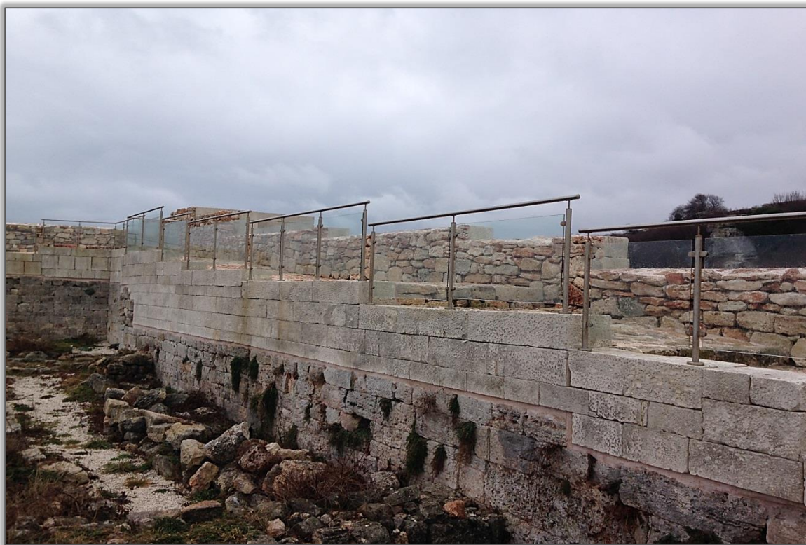
Fig.8. Staircase after the restoration, showing the difficulty to observe evidence for the original height or length (photo by the author).
