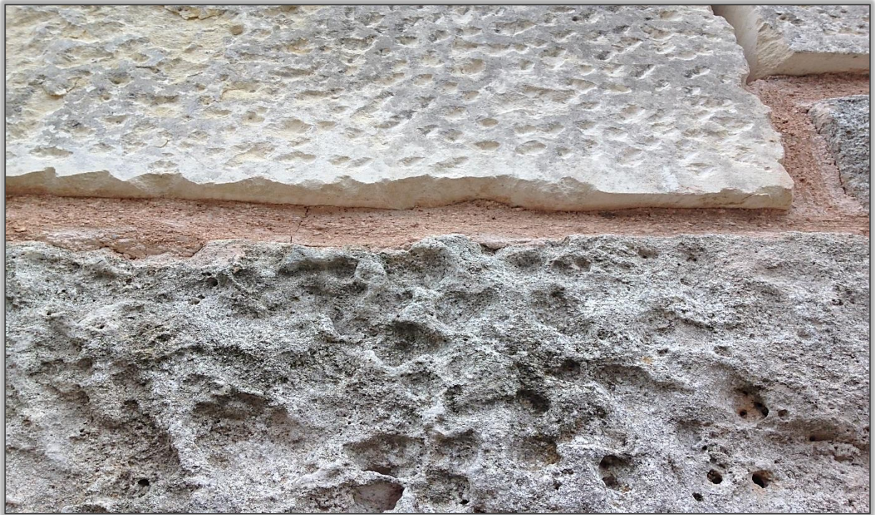
Fig. 10. Observing the distinction between the new and authentic fabric (photo by the author).
