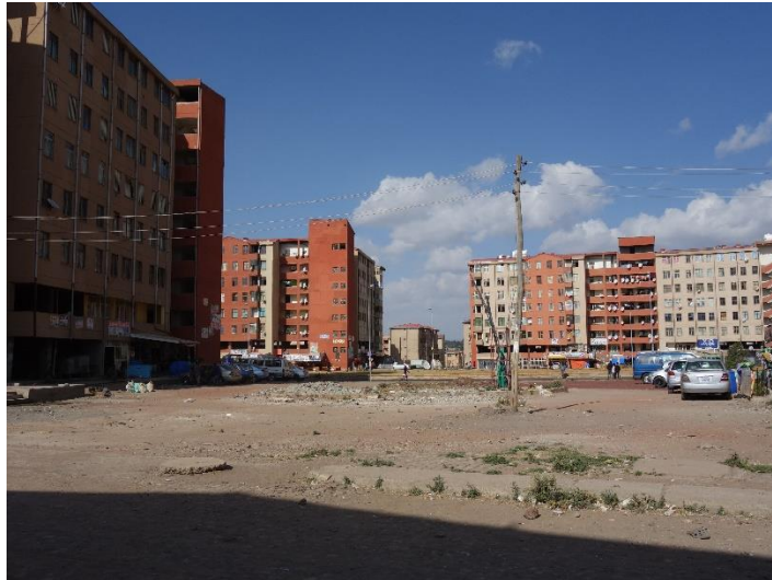
Arabsa condominium blocks (2020)
