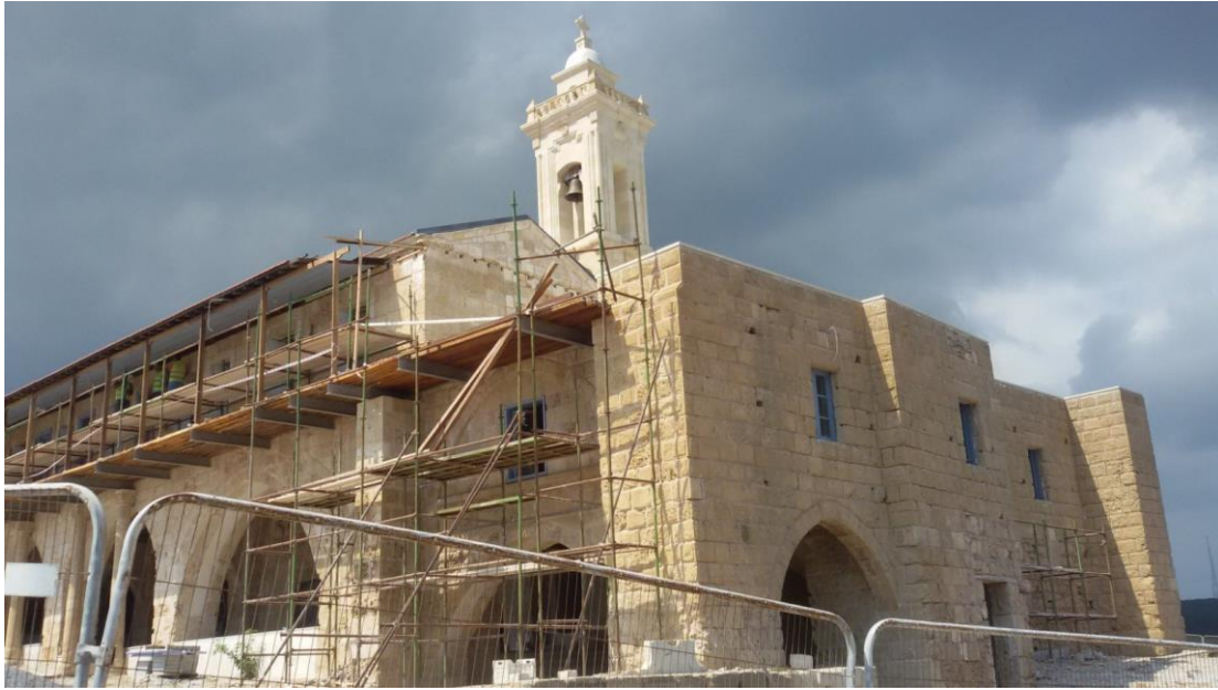
Figure 8. Restoration works in progress (2016). Photo by the author.
