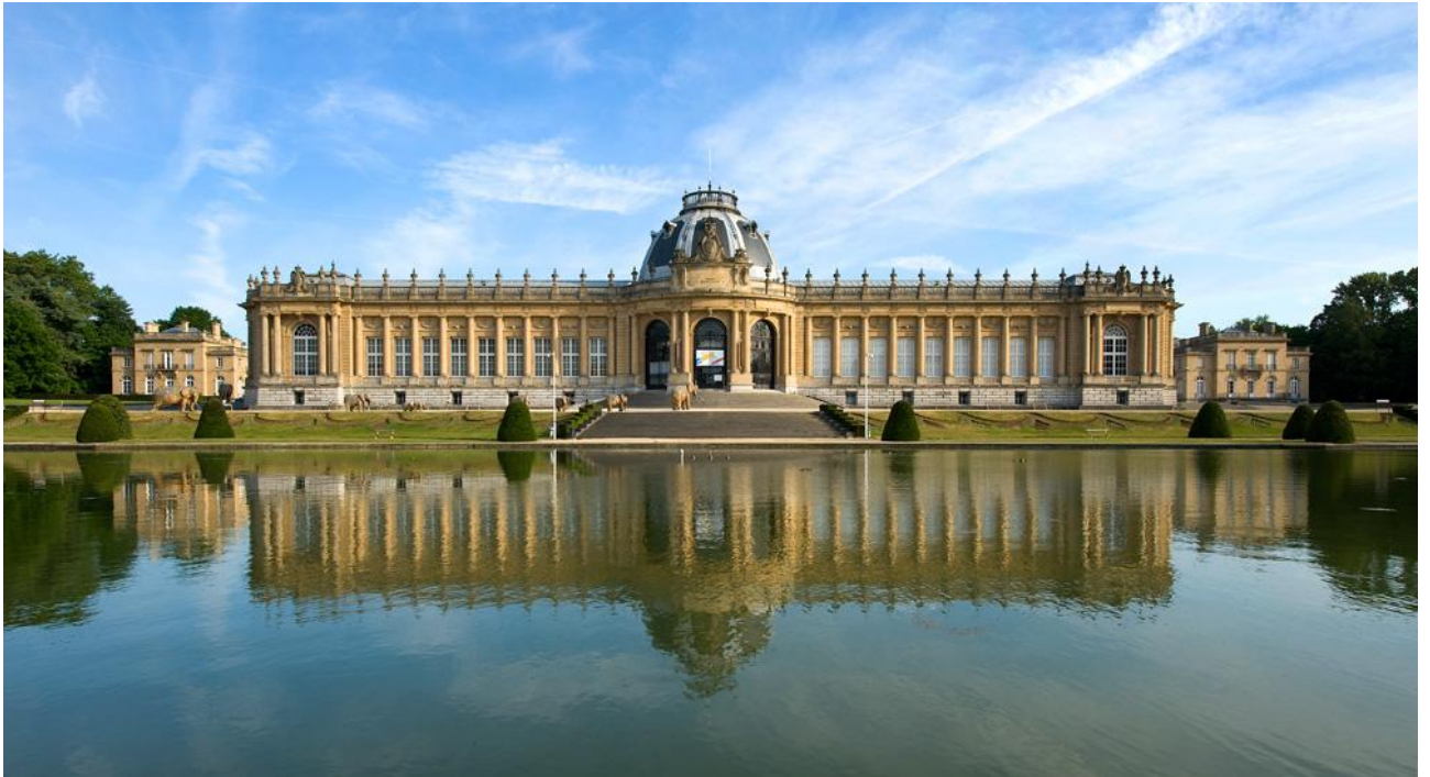
Fig. 1.1: View of the main building of the Royal Museum for Central Africa.
