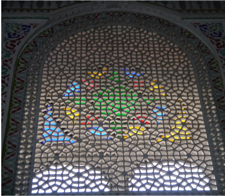
Figure 51: Lattice from the mehmonkhona in the Abram Kalontarov house. Note the coloured stain-glass behind the Bukharan-style lattice ( panjara ). (Photo by author).
