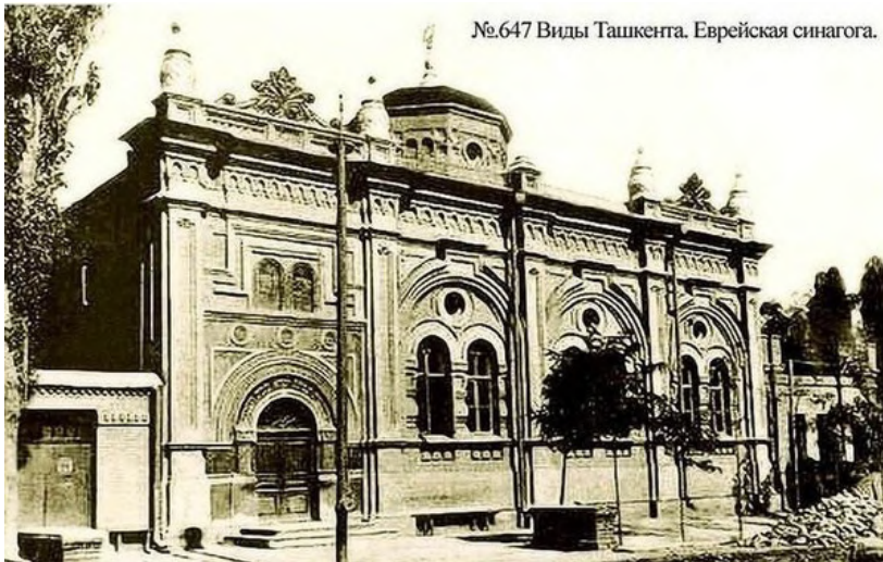
Figure 86: Drawing (a) and photograph (b) of the Ashkenazi synagogue in Tashkent. (The Center for Jewish Art).
