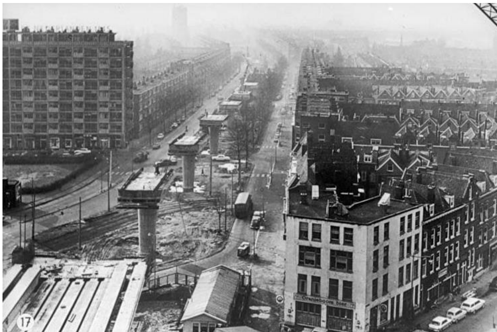
Image 1, the construction of the metro line through Mijnsheerenlaan around 1965. 26
