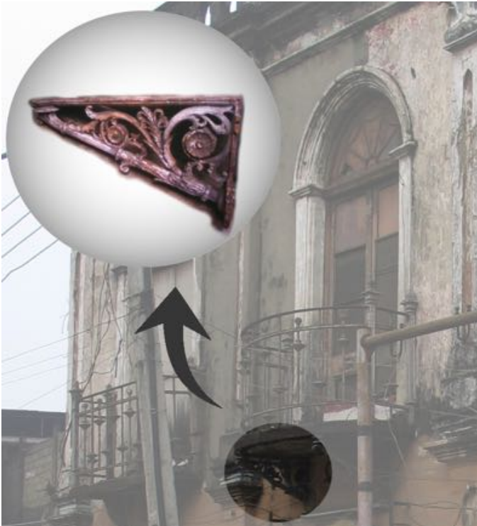
Illustration 4: The balcony bracket that was for sale after the demolition (source: Ktravula.com) showing where this architectural element used to be. (Source: Legacy)
