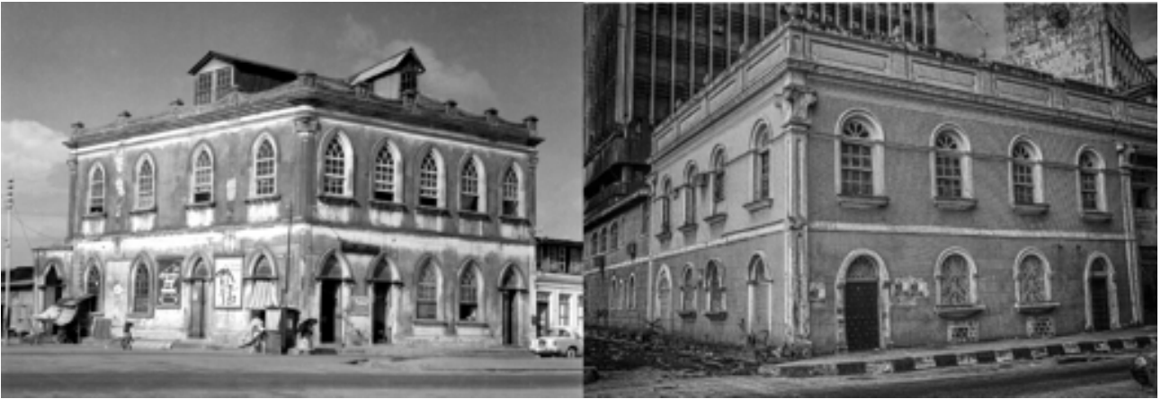
Comparing two Brazilian style buildings on Lagos Island: on the left Araromi House, on the right Water House (Source: Wikimedia Commons)
