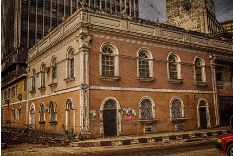
Water House on Kakawa Street, Lagos Island, in 2016 (Source: Wikimedia Commons, photographer: Arafat Awoyejo)
