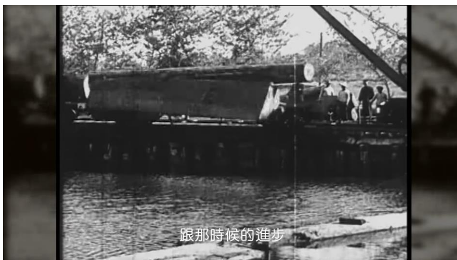
Figure 15 “The advancement of that period (birthed the most extensive national sawmill of the Japanese Empire)”. (Source: The Heart of the Alishan Forest Railway )
