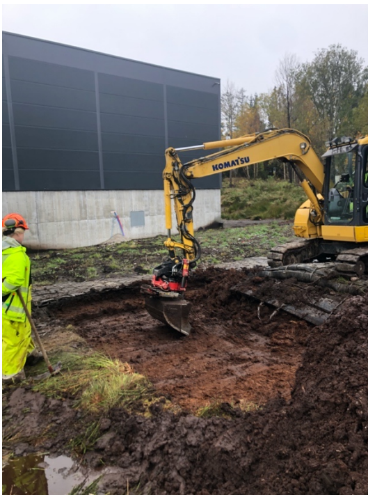
Figure 6: Haraldstadmyr excavation, November 2020.
