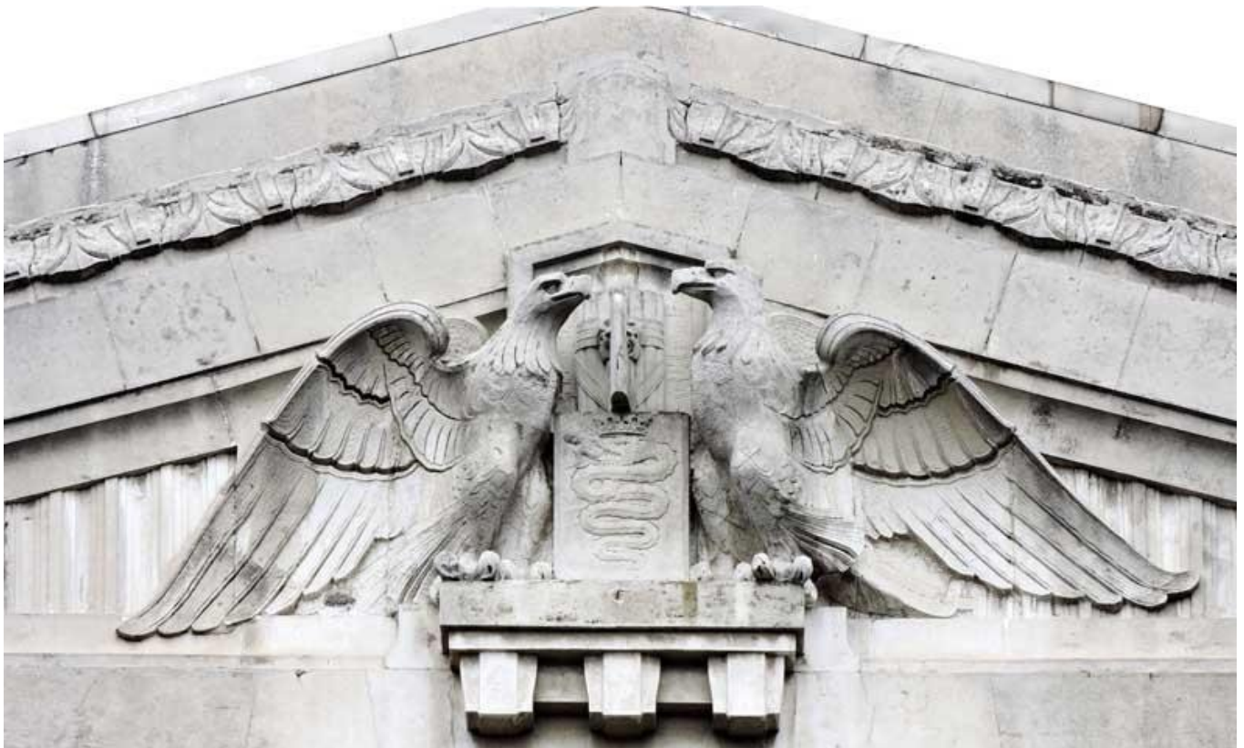
Figure 11: Milan station detail
