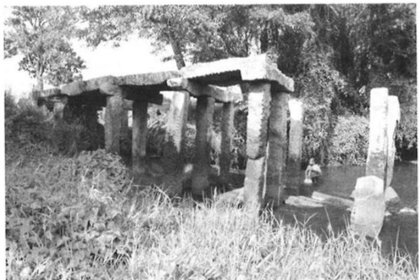
Figure 67. A stone bridge across the Malwatu Oya
