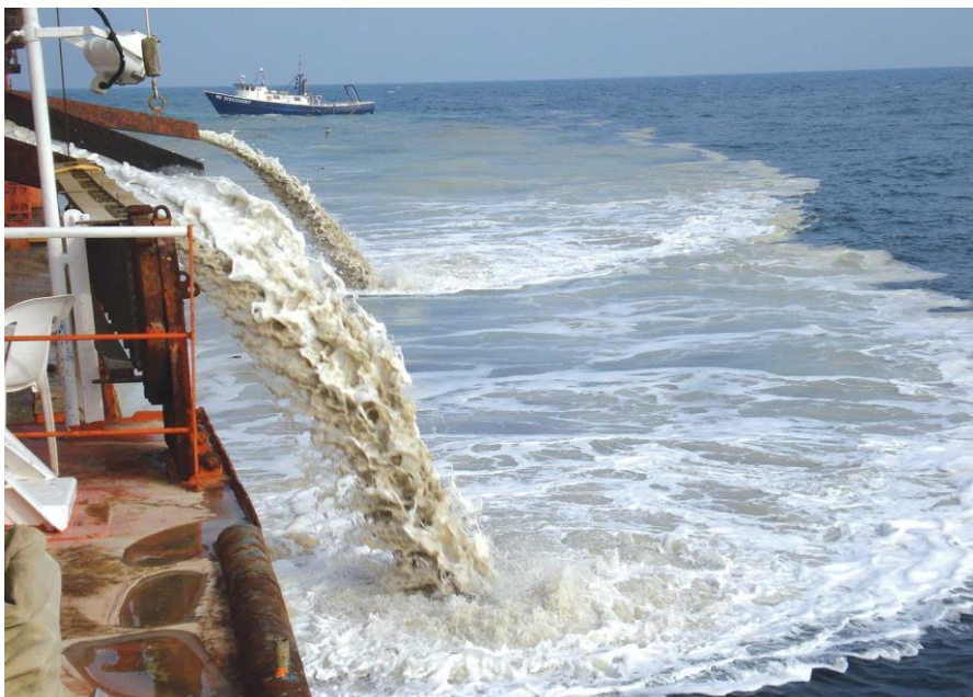
Figure 4.9 – Release of excess water from the hold during the extraction process, which leads to the formation of density plumes (iadc-dredging.com).
