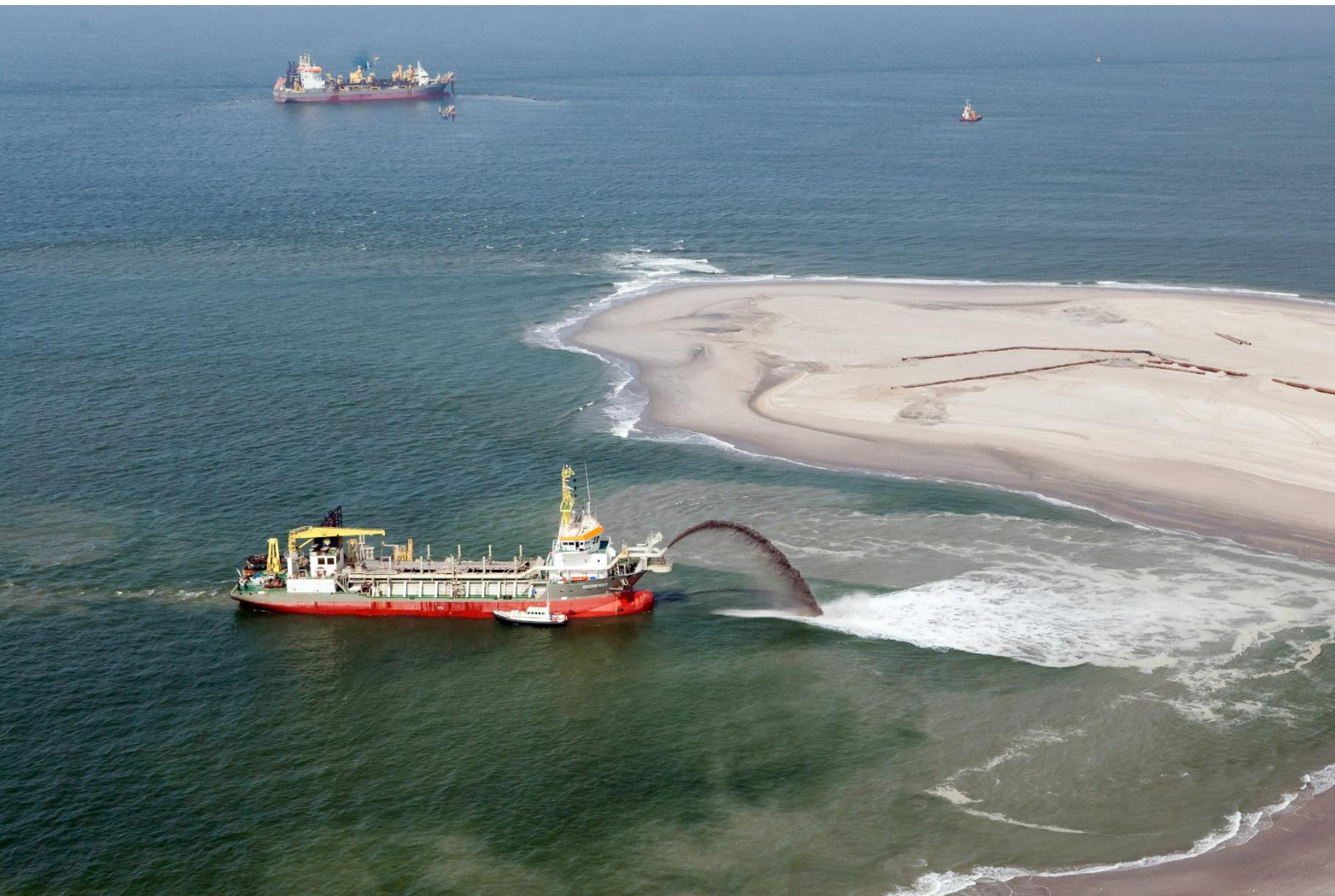
Figure 4.1 - The process of 'rainbowing' sand during the construction of the Sand Motor (Zandmotor) at the beach of Monster, Zuid-Holland, in 2011 (beeldbank.rws.nl).
