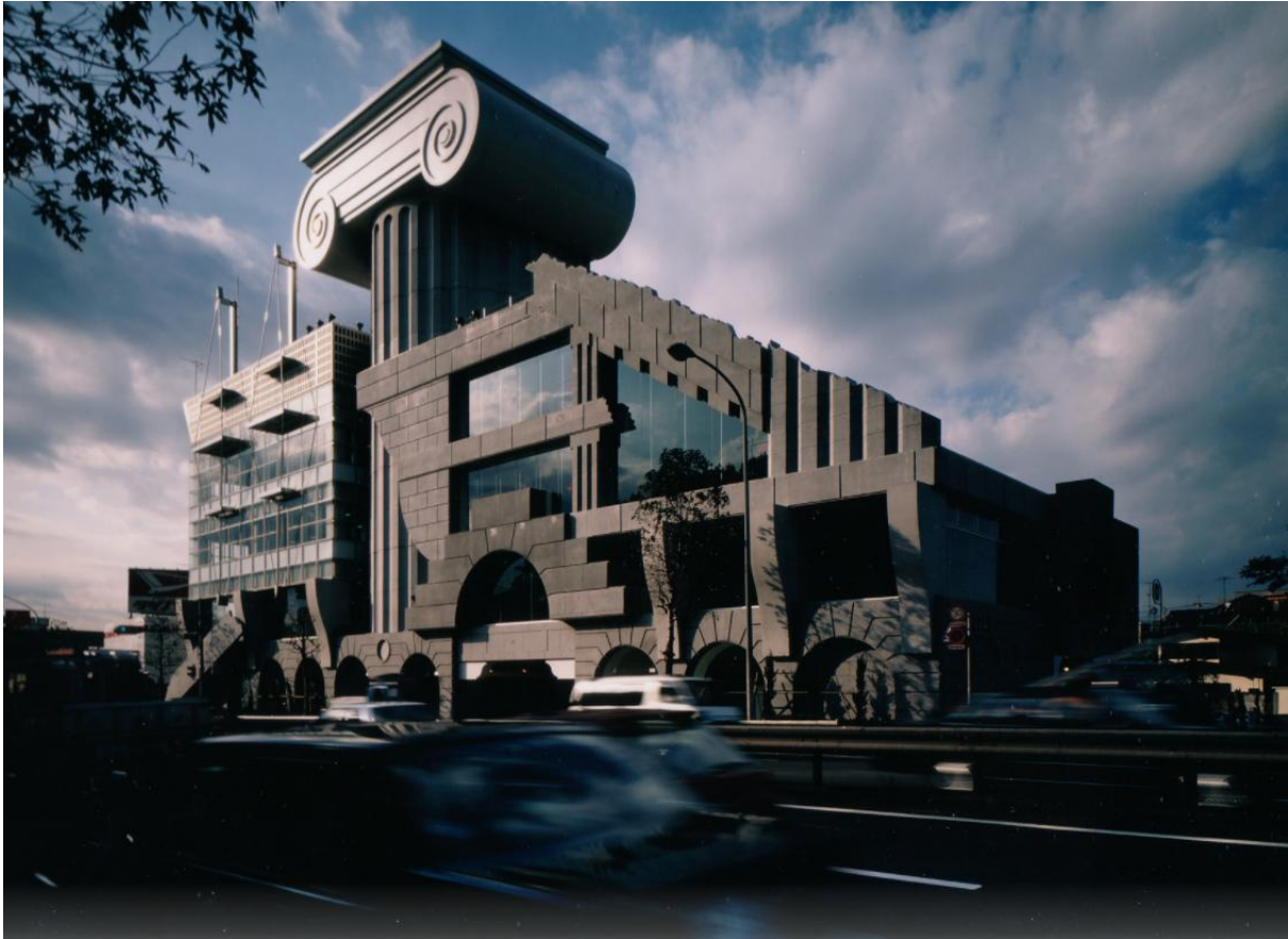
Figure 2. The M2 building (Source: Kengo Kuma and Associates)
