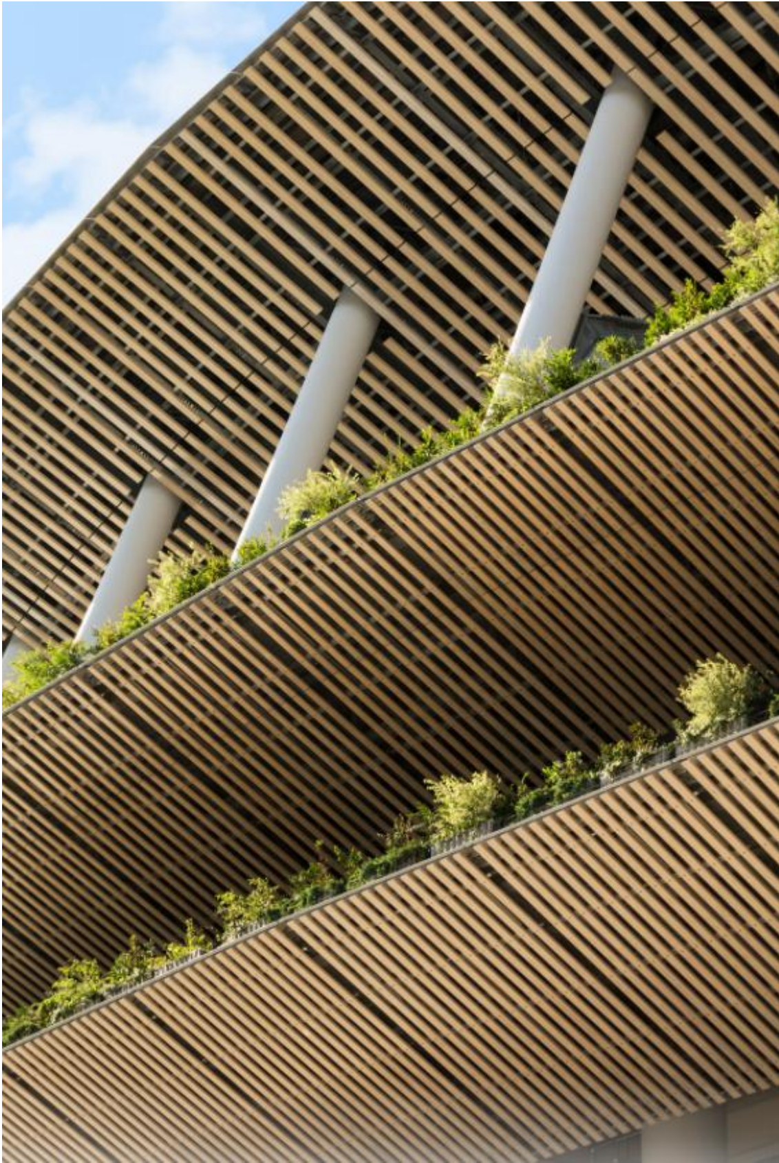
Figure 5. Utilizing Plants to Blend the Olympic Stadium with the Surrounding Park (Source: Kengo Kuma and Associates)
