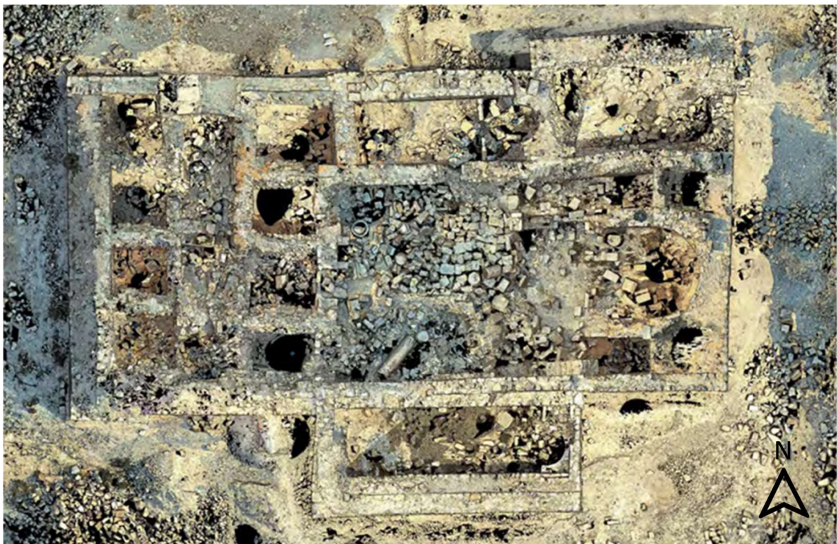
Figure 2.2: Top plan of Udhruh church from Al-Bashaireh, K., Abudanah, F., & Driessen, M. (2020). Provenance analysis of marble ecclesiastical elements from the extra-mural Byzantine church of Udhruh (South Jordan) p. 4.
